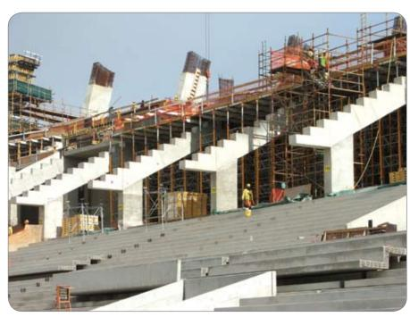
Fig. 7: Raked beams on which the 20 ton precast seating elements will rest.
