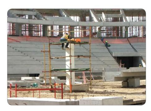
Fig. 6: Checking the placing position of the precast seating elements from a 4 m high pillar on the future pitch.
