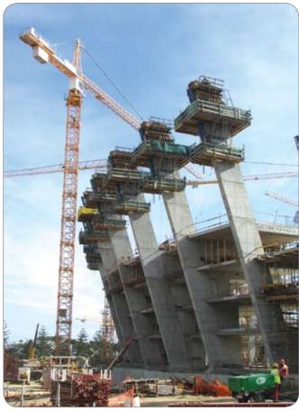
Fig. 5: Construction of the pylons is being done in lifts of 3,8 m. For each lift the formwork has to be positioned correctly.
